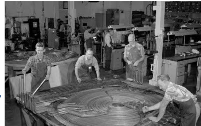
Building the 88-Inch Cyclotron. Internal cooling water lines are shown.
