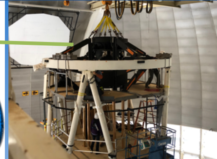
12-ton corrector installed Nov '18
