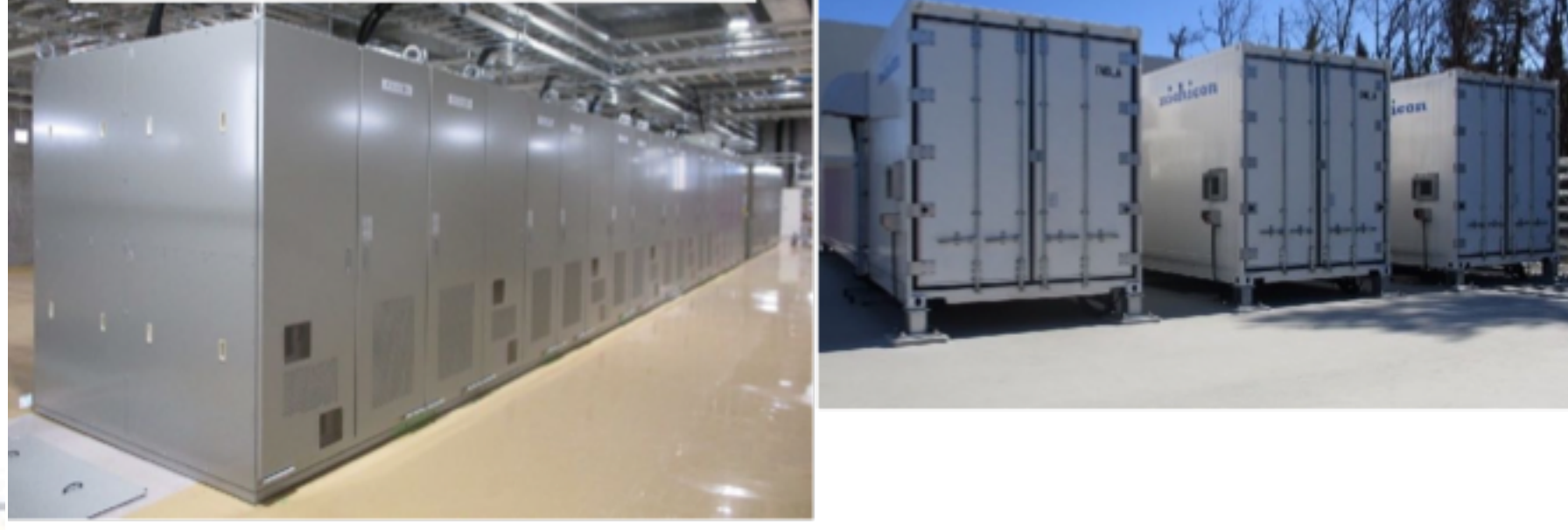
New main magnet PS for high rep. rate
